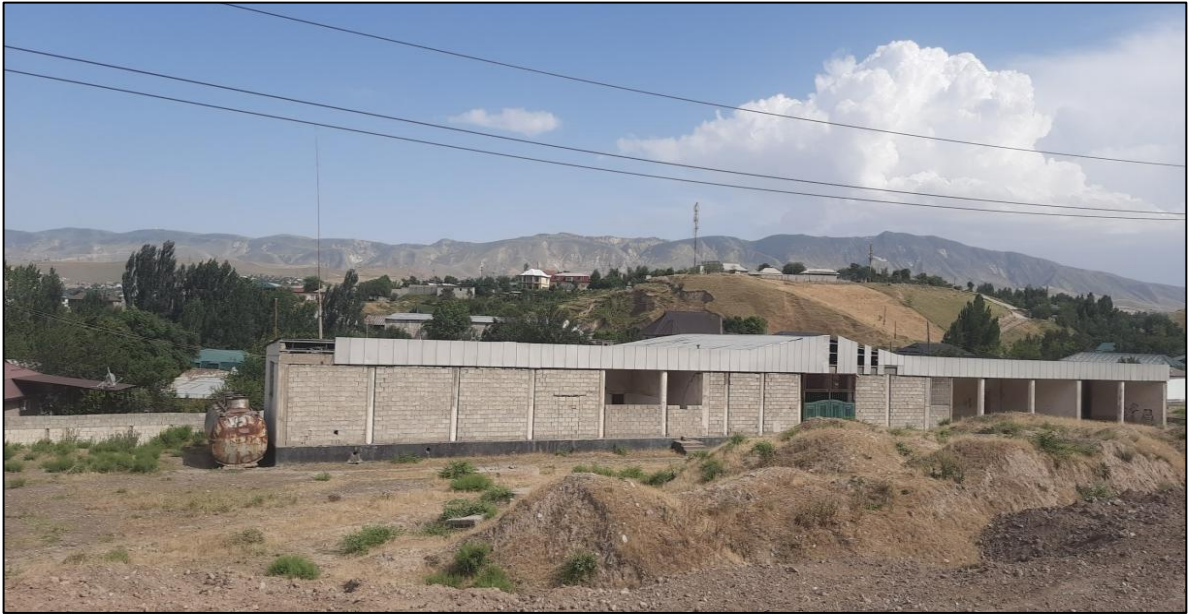
No 1. Photo of adjacent land parcels and unfinished structures located at km 7+350 - km 7+645 LHS of Dushanbe -Kurgonteppa Phase 1 road section and covered under the CAP (original condition).
