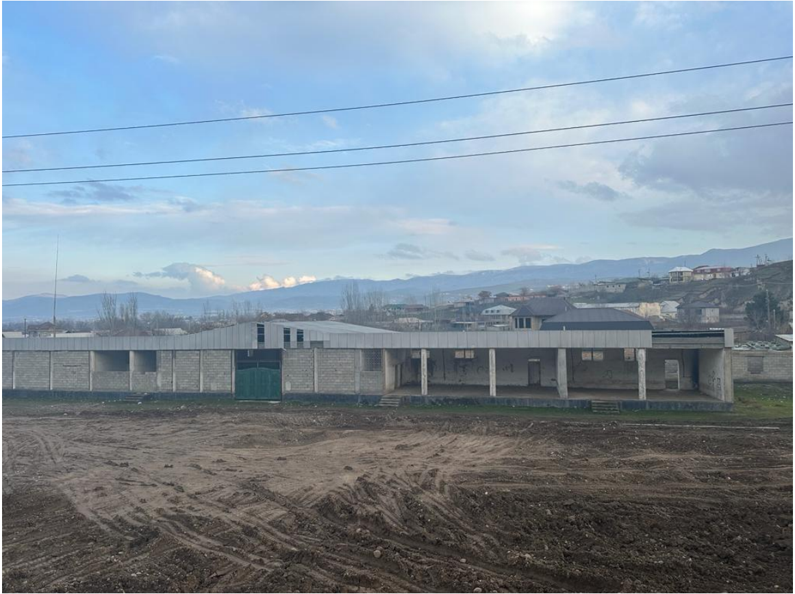
Photo No 3. Contractor levelled the piles of soil as requested by the owners.
