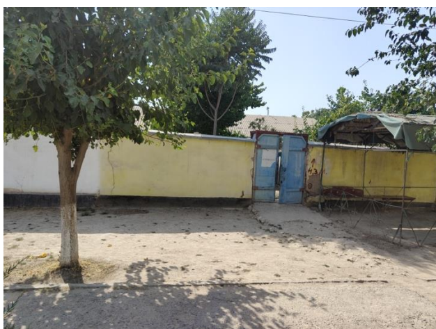
Affected boundary structure
