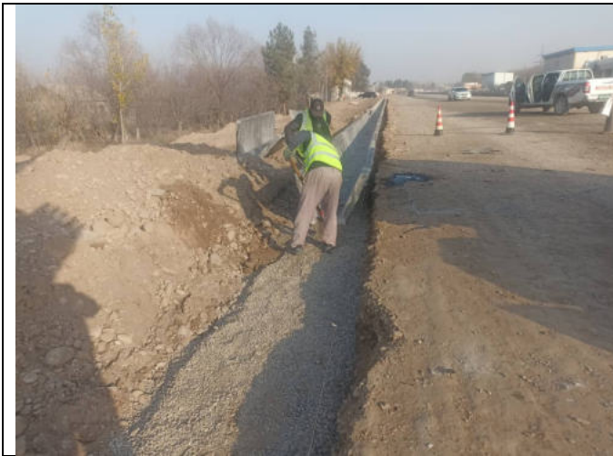
Installation of L2-1 trays and PP-1 slabs
