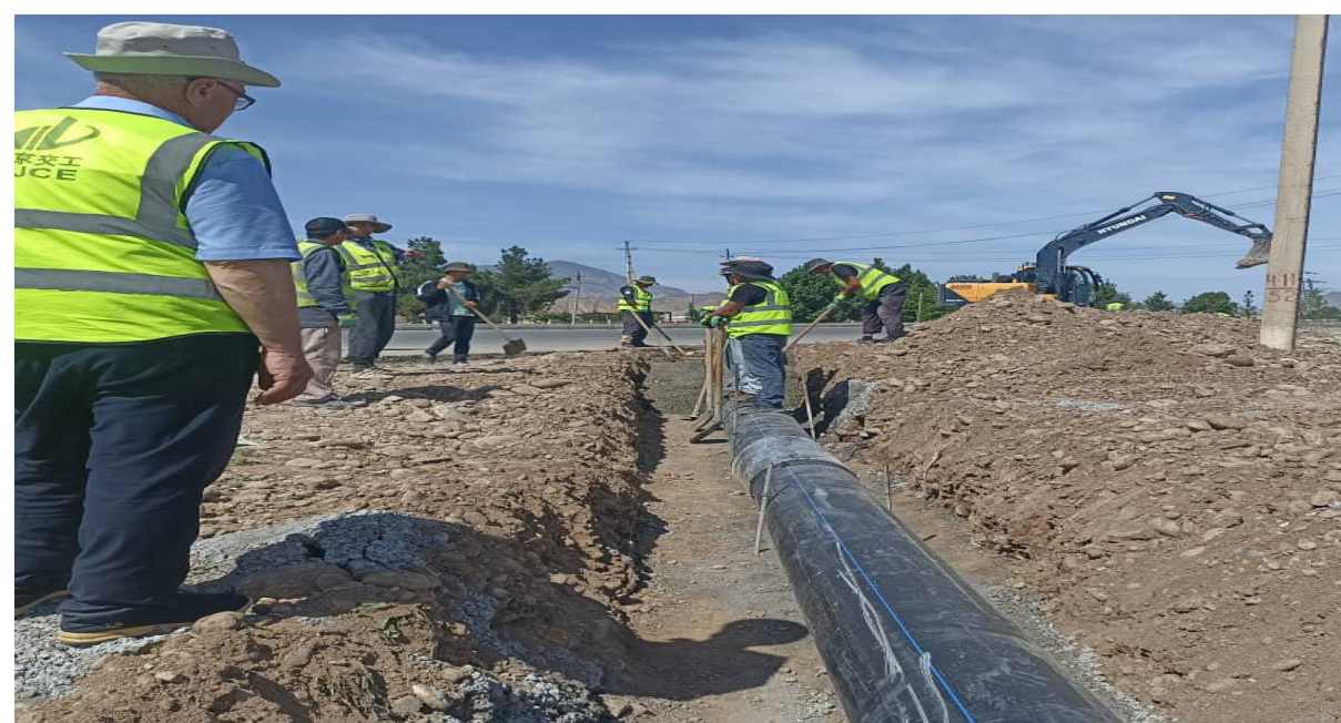
Laying a polyethylene pipe for draining water into the canal and concreting the pipe cavities on the right side of the road
