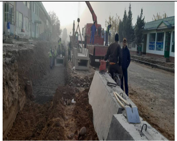
Installation of L2-1 trays and PP-1 slabs
