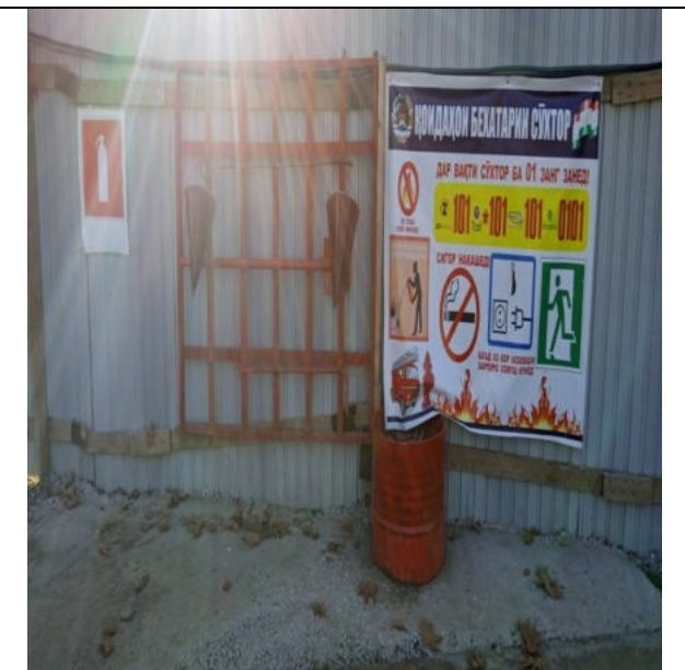
Photo. Fire shields.
