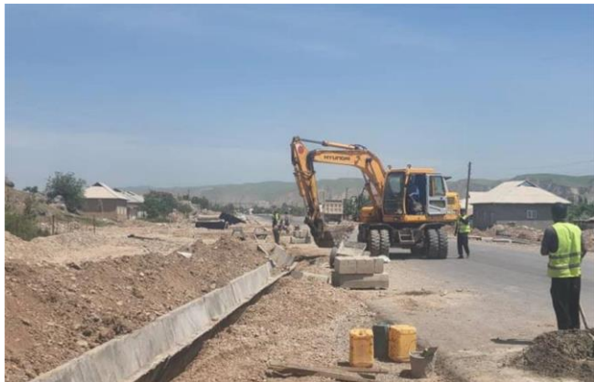
Photo 13: Installation of drains, May 2023
