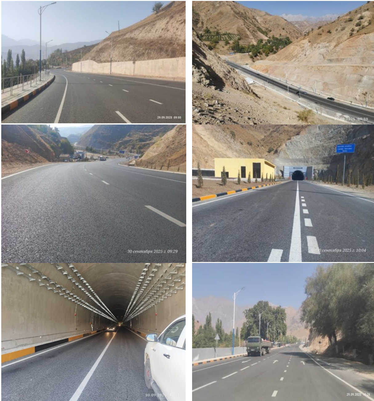
Inspection to the project road. The completed Obigarm-Nurobod road project inspected in September 2025.
