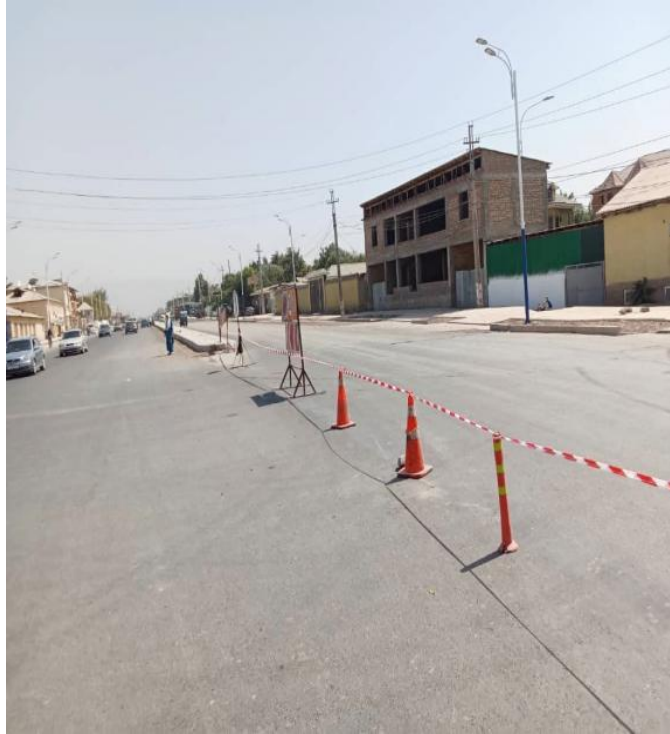
Asphalt paving of the road km 9+720 08/23/2024.
