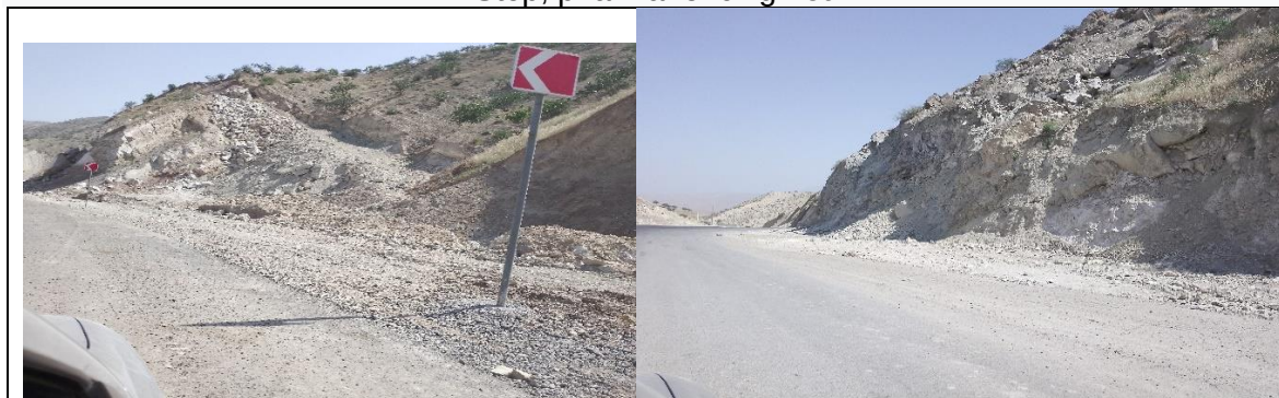
Place of construction of the road object lot-2
