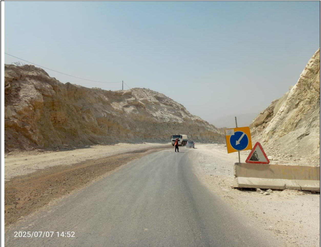
Performing works to eliminate collapse
