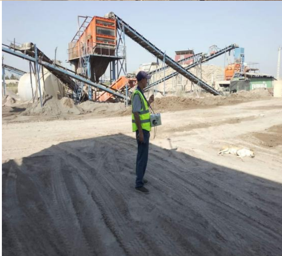
Watering to control dust and Monitoring Air Quality
